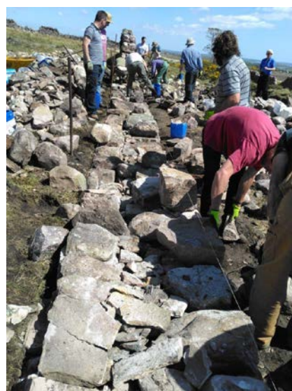
Repairing Stone Walls on the Greenway
