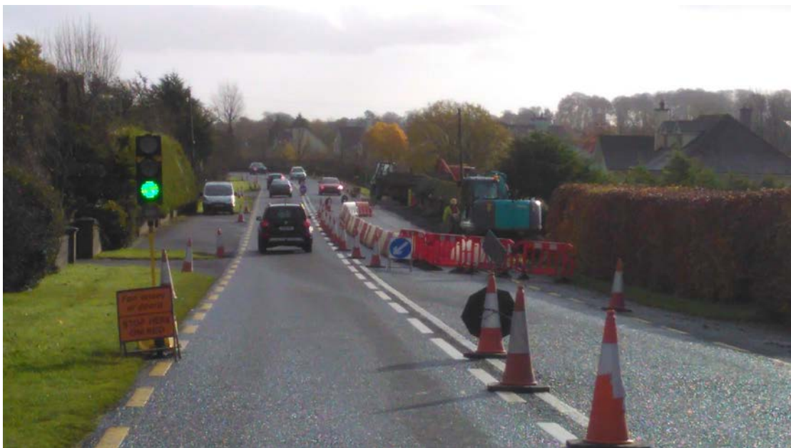
Breaffy Sewerage Scheme in progress
