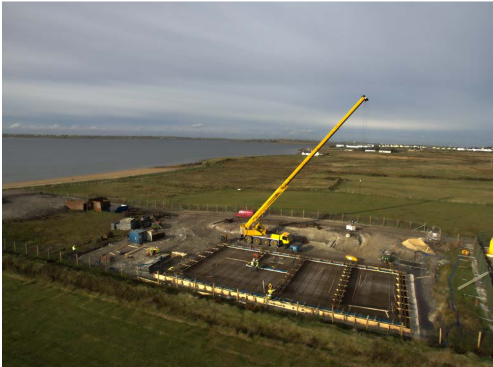
Belmullet Sewerage Scheme (Wastewater Treatment Plant under construction)
