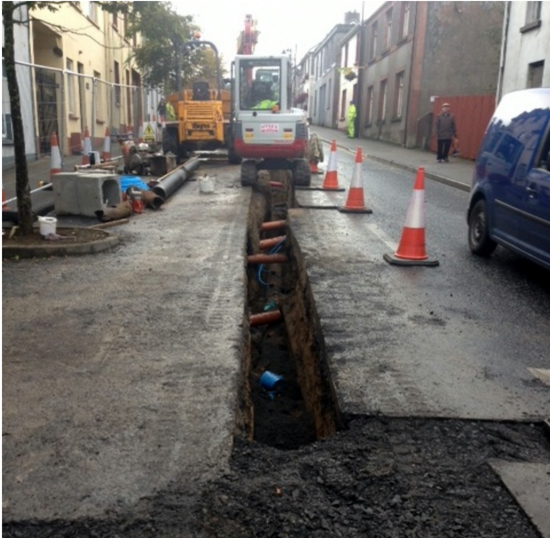
Ballina Mains Replacement Works
