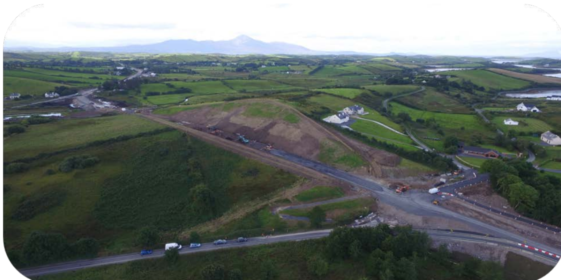
N59 Rossow Bends Construction works
