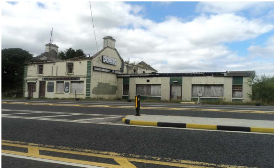
Derelict Site Before Demolition – Ballyvary, Co. Mayo
