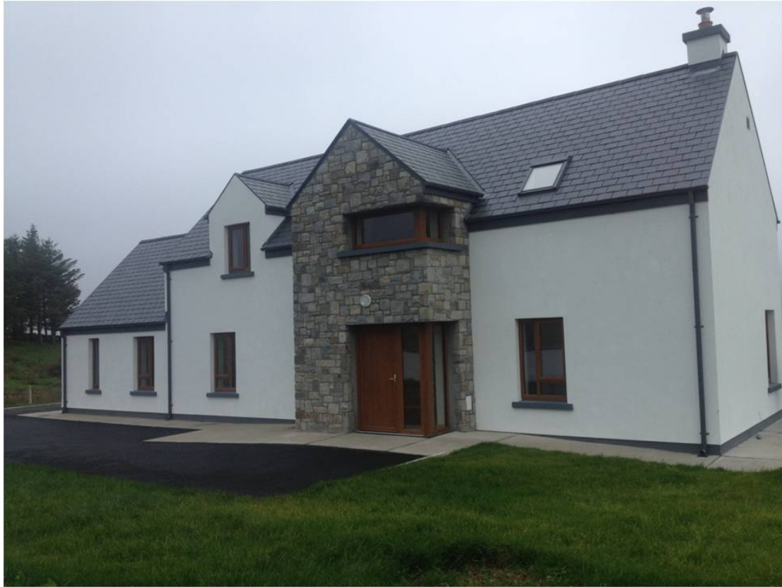
4 Bedroomed Single Rural House Type - 5 Currently under Construction
