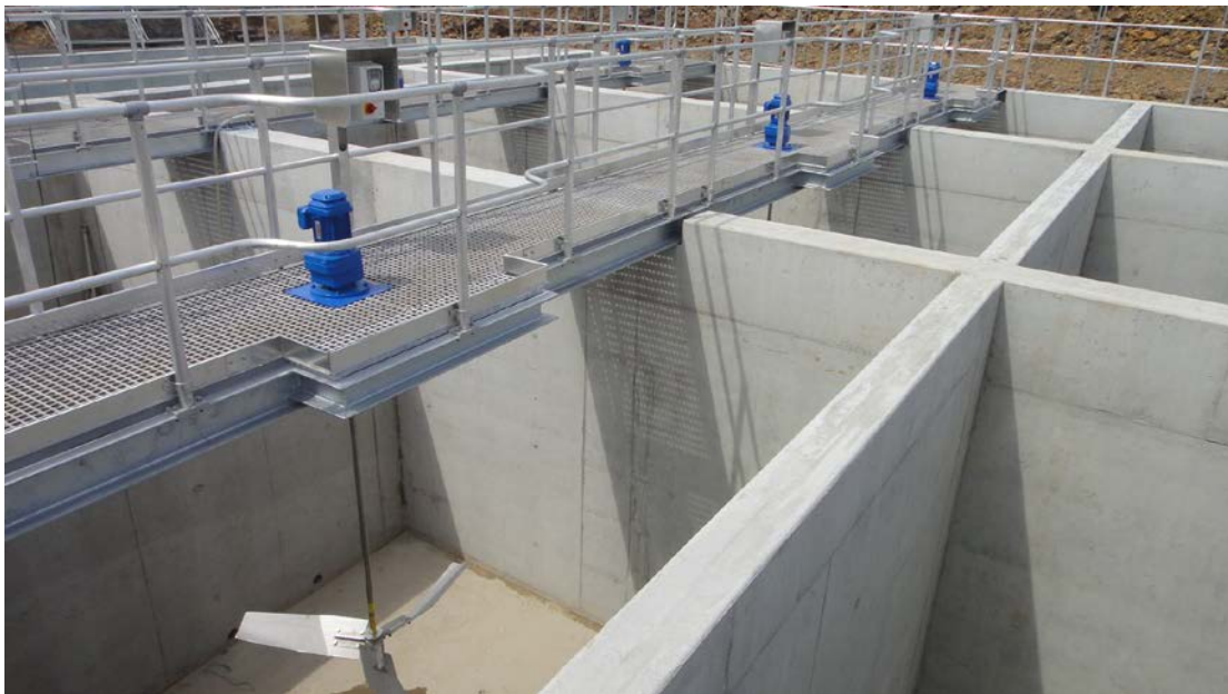
Upgrade works at Lough Mask Water Treatment Plant
