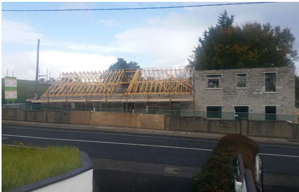
Marian Crescent, Ballina - Infill Site - 4 Units Under Construction
