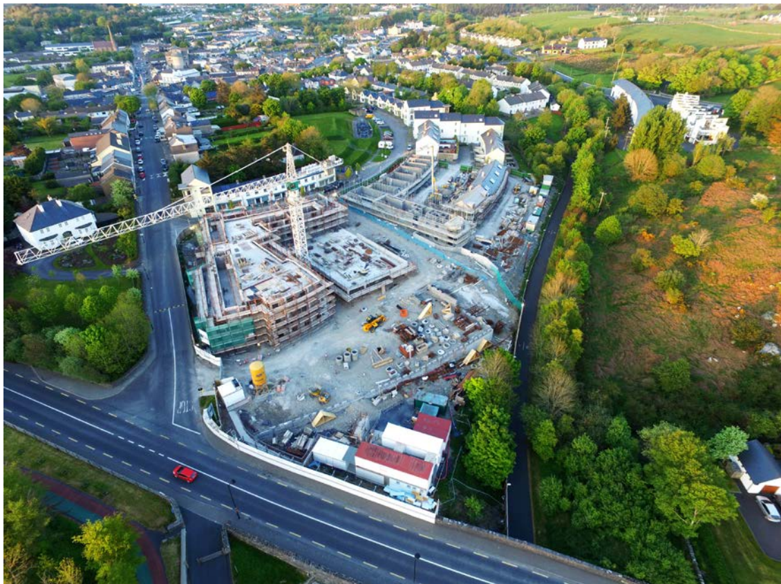
Tubberhill, Westport – 21 Housing Units under Construction
