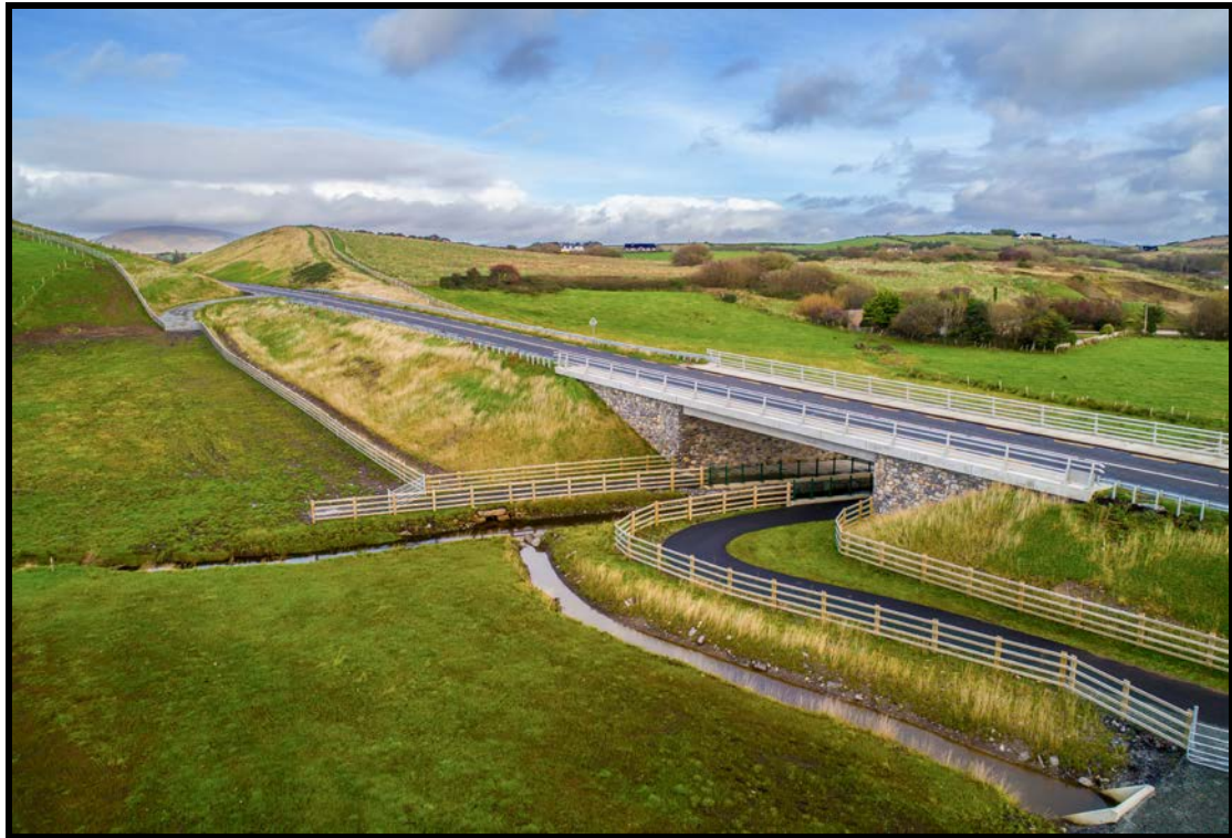
N59 Rossow Bridge
