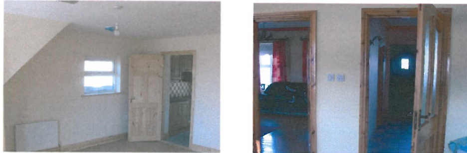
Long term Voids – Pre Letting Repairs
