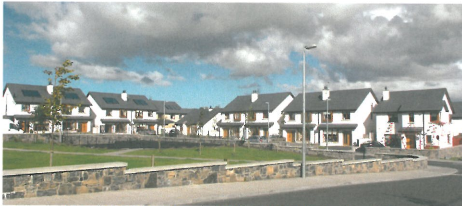
St Patricks Estate, Ballina – CLSS – Cluid Housing Association
