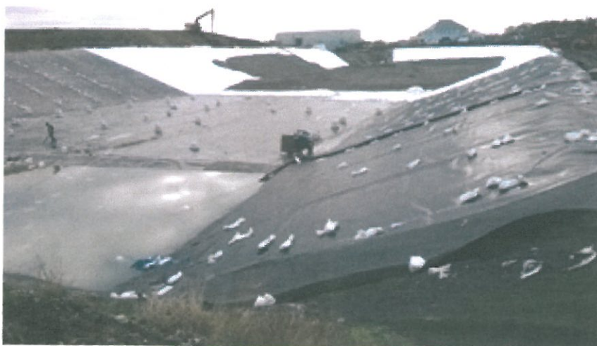
Leachate Drainage layer being put on (top of picture)
