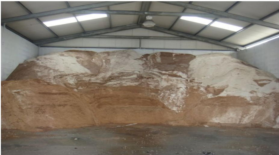
Figure 5: Salt storage barn
