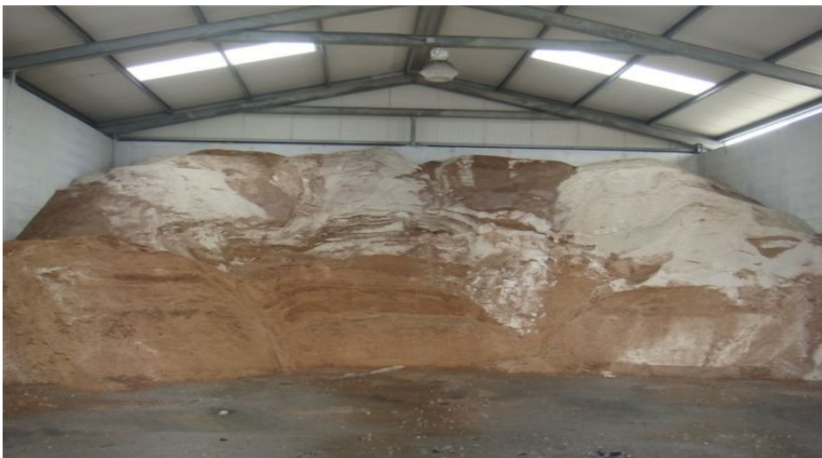
Figure 5: Salt storage barn
