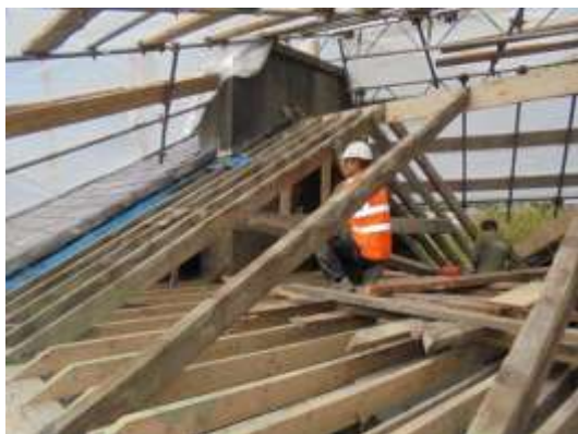
Roof reconstruction with original rafters & collars
