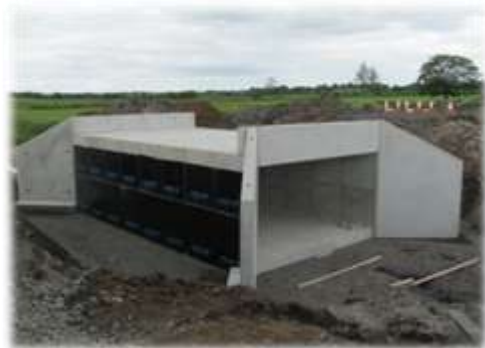
Placing of culvert sections
