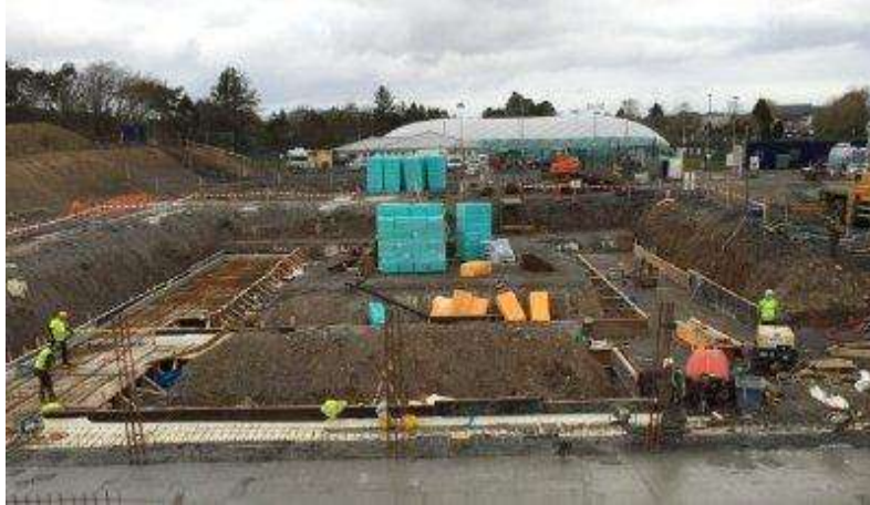
Construction on site
