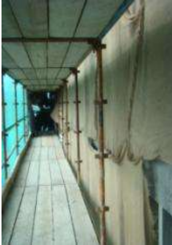
Hessian protection to lime works
