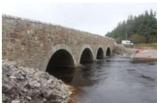
Mount Jubilee Bridge Widening Scheme
