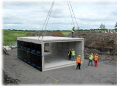
Kilnock Bridge newly constructed
