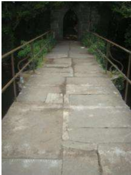
Footbridge, Cong: Before
