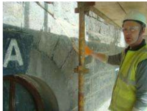
Lime mortar pointing
