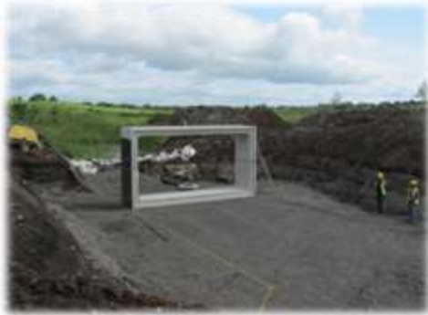
Kilnock Bridge prior to construction
