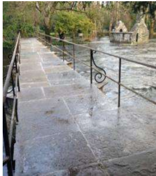
Footbridge, Cong: After
