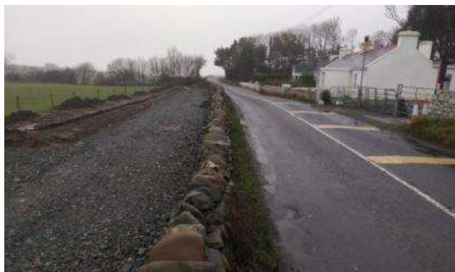
Lecanvey Improvement Scheme under construction
