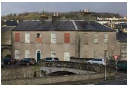
Bridge House, North Mall, Westport: Before
