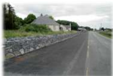
Overall View of Works at Robeen Church
