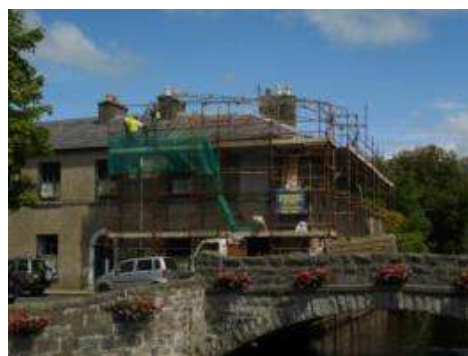
Bridge House Scaffold
