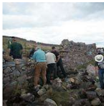
Repairing Stone Walls on Greenway, Mulranny
