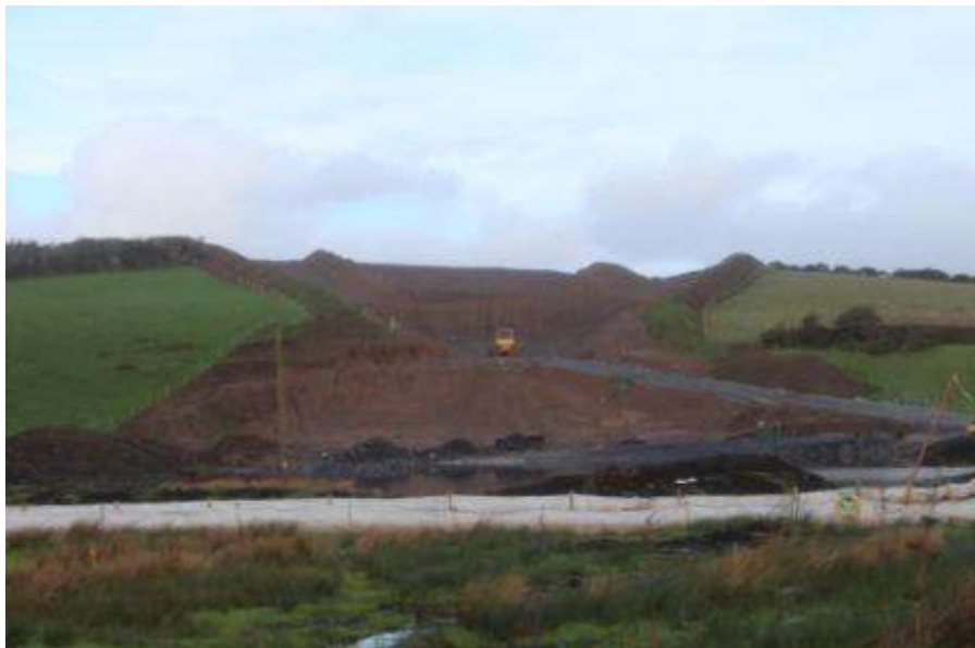
N59 Rossow Bends under construction
