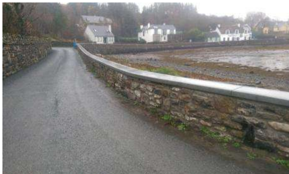
Rosbeg Wall Repairs
