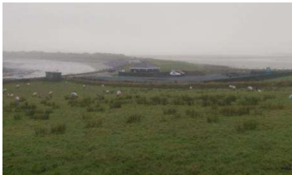
Bertra Car Park under construction
