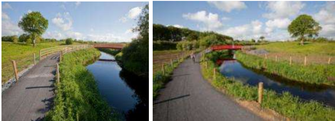
Castlebar to Turlough Greenway
