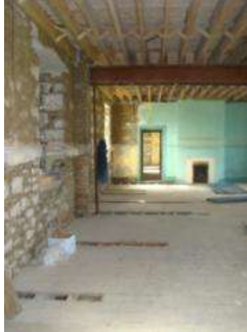
Drying out to walls & timber treatment
