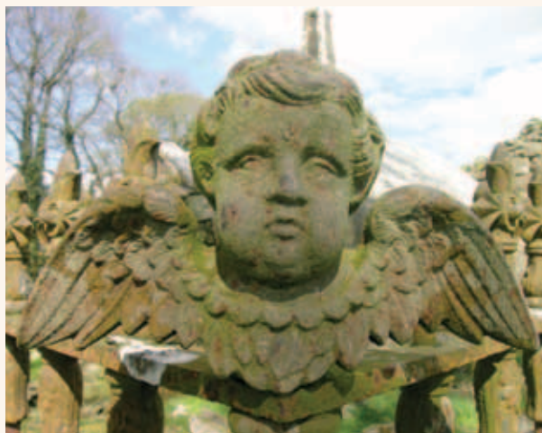
This cast iron cherub on the railing of a burial plot at Tulske, Co. Roscommon, is in need of basic conservation work
