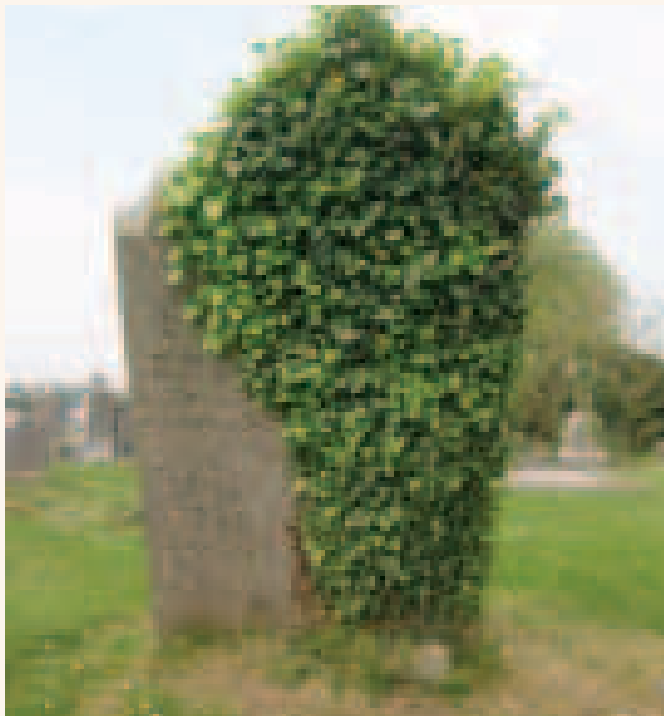
Weedkiller has been sprayed around the base of this headstone allowing the ivy to thrive
