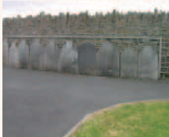
At this graveyard, memorials have been removed from their original location and placed against a graveyard wall. The heavy ribbon pointing of the graveyard wall should also be avoided
