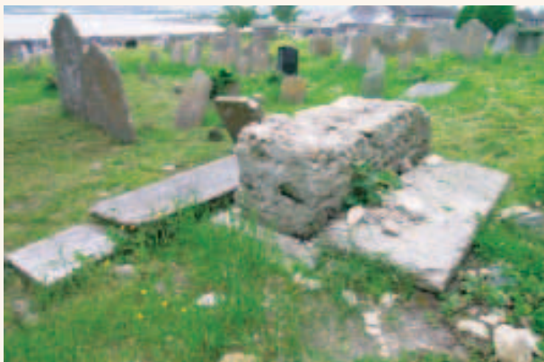
This vandalised chest tomb is in need of basic conservation work
