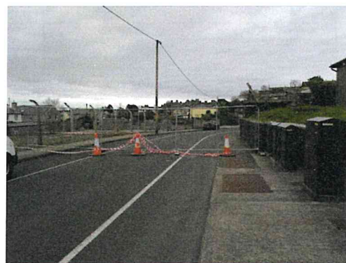
Following a fire at the former Duffy's bakery in Ballina, debris from the Asbestos roof was dispersed in the adjoining area. An Asbestos clean up of James Connolly St was completed by specialists and the street closed.
