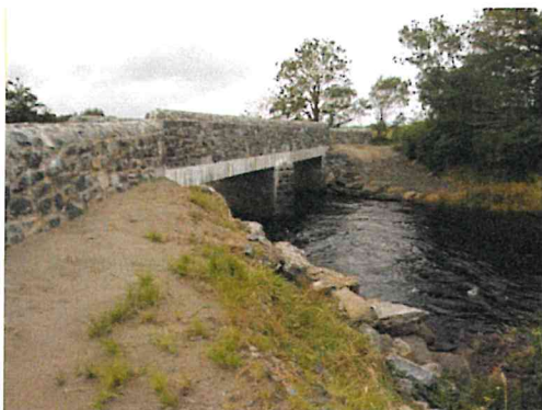
Ferrew Bridge reconstruction
