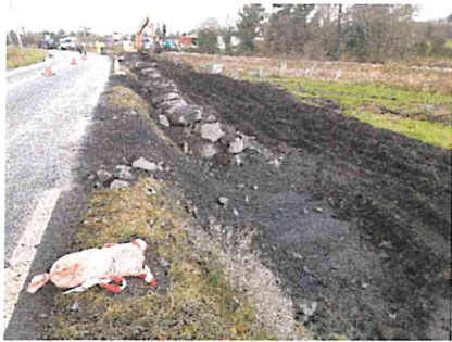
Road widening at Behy
