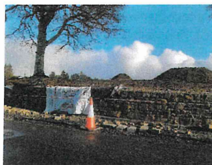
Community Involvement Schemes at Attymass Rd, Bonniconlon which included road widening, new footpath and stone wall.
