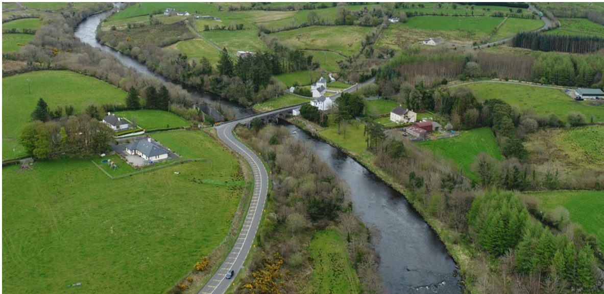
N26 Cloongullane Bridge, Swinford
