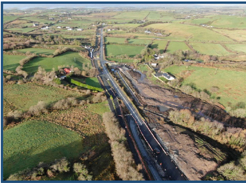
Works underway on the N59, at Kilmeena.
