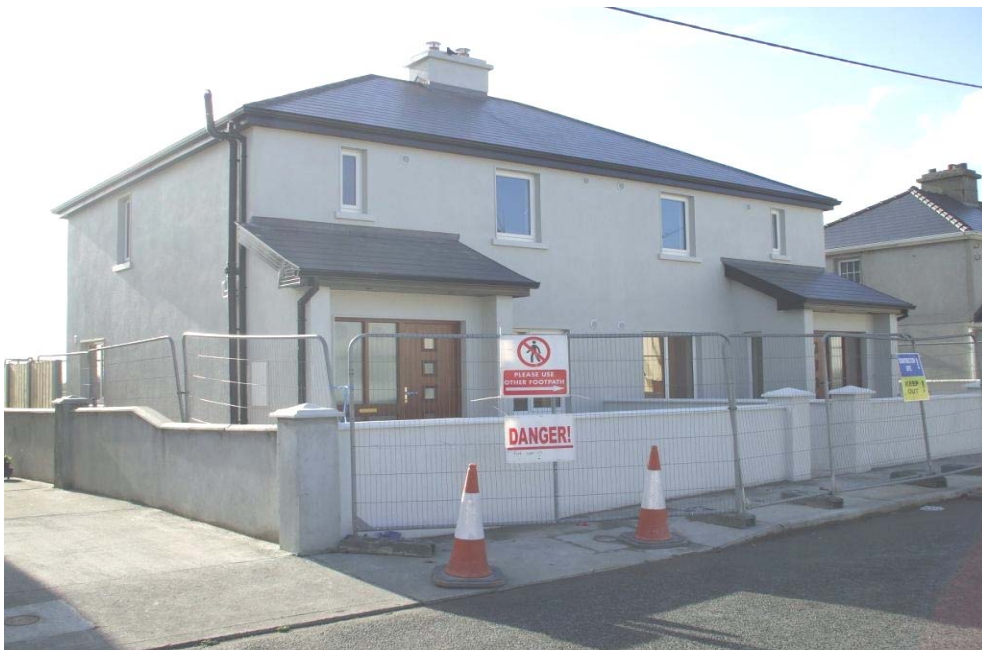
Roches Terrace, Ballina – Development nearing completion
