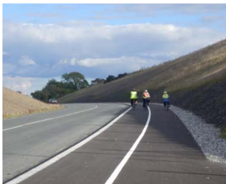
Segregated Walking and Cycling Trail along the Newport Road, Castlebar
