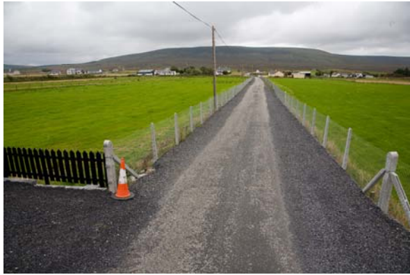
Glenamoy Road Upgrade
