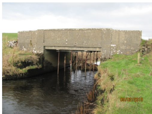
Kilknock Bridge (Before Works)
