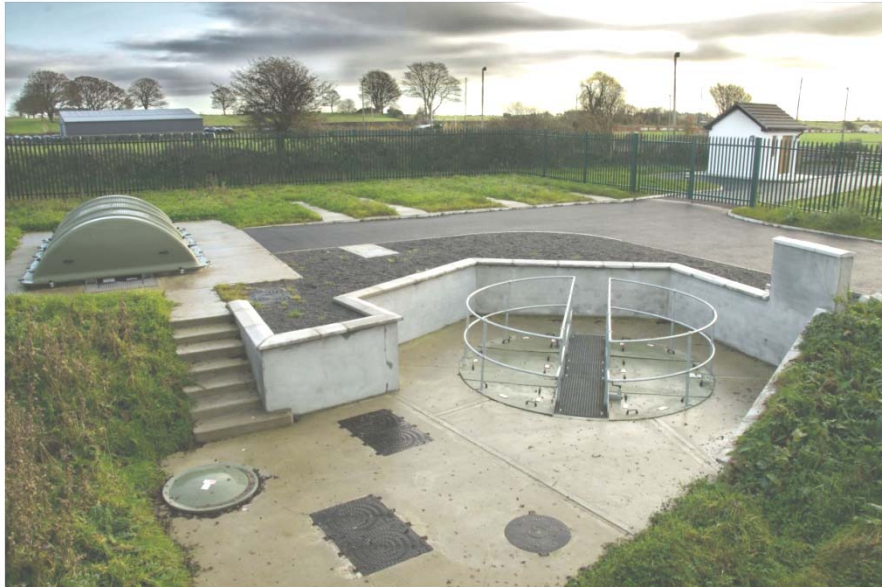
Mayo Abbey Sewerage Treatment Plant
