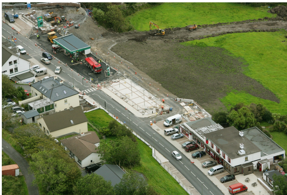
Improvement Works in Progress in Mulranny in 2015
