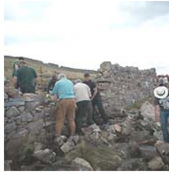
Repairing Stone Walls on Greenway, Mulranny
