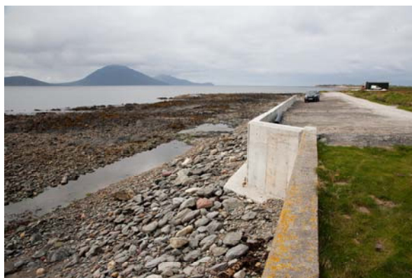
Storm Damage Repair, Doohoma Pier, Belmullet
