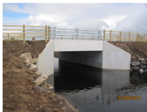
Kilknock Bridge (After Works)
