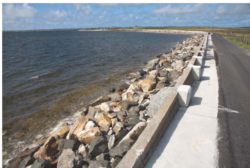
Storm Damage Repair, Ardmore, Belmullet
