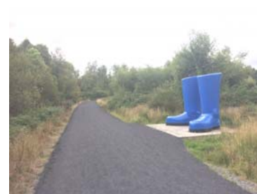
Completed Works on the Land of the Giants Greenway, Claremorris
