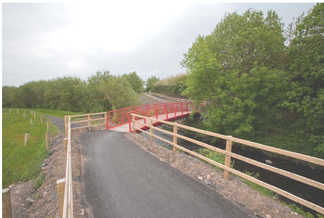
Castlebar – Turlough Greenway
