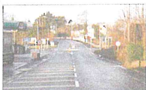
Sligo Road Roundabout
