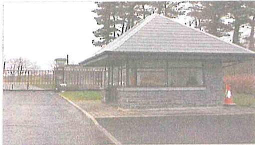
Initial Incident Control Point - Gatehouse
