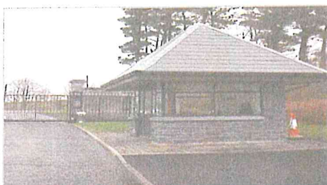
Initial On-Site Co-ordination Point - Gatehouse
