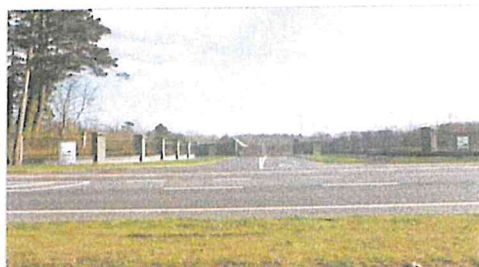
Holding Area 1 – Entrance Gate to Atlantic Industries
