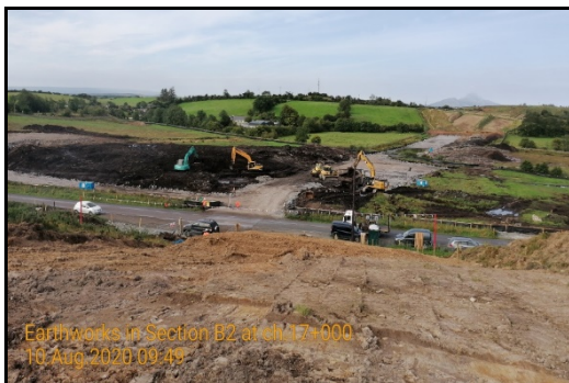
N5 Westport to Turlough Road Project-Works at Islandeady Road
