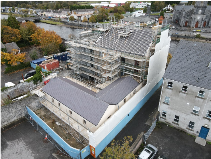
Mary Robinson Centre making good progress on site.
