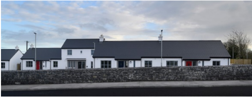
Recently Completed Parke Housing Scheme
