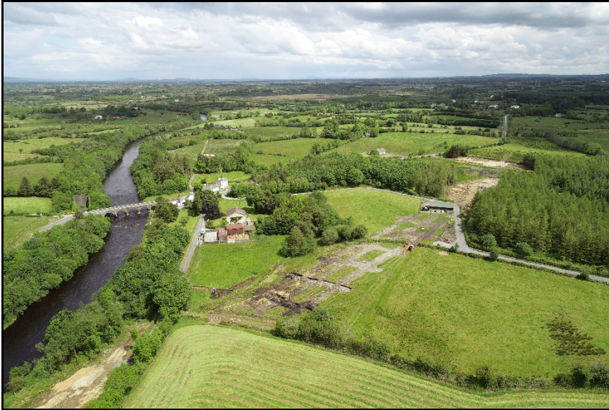
N26 Realignment at Cloongullane Bridge-Archaeological Trenching
