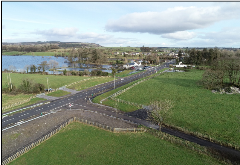
N60 Lagnamuck Scheme-Substantially Complete
