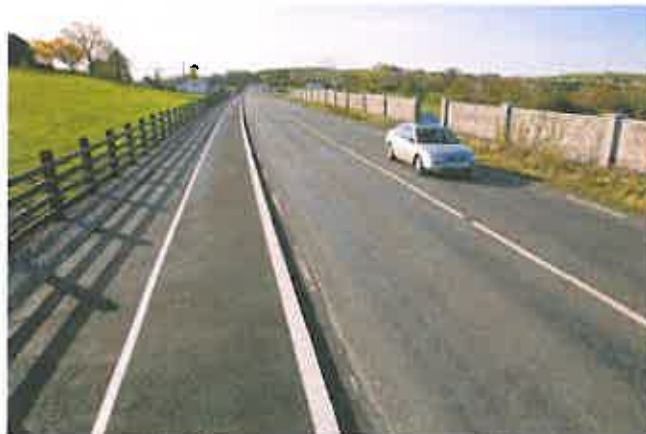
New Greenway, Newport Road, Castlebar
