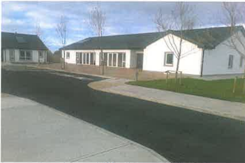
Community Building – Mayfield, Cluremorris – CLAR ICH
