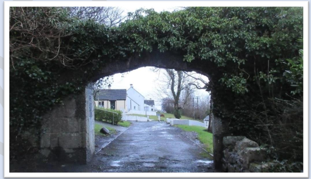
Fig. 34 A former entrance to Newport House demesne, Newbridge Street, 2018
