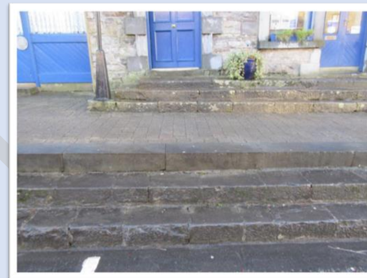
Fig. 32 Limestone steps, Main Street, Newport, 2018
