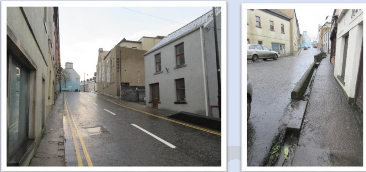
Fig. 50 Footpaths, George's Street, Newport, 2018
