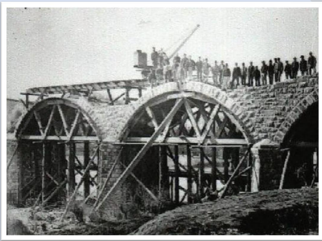
Fig. 15 Newport viaduct under construction, c.1890 ( www.askaboutireland.ie )
