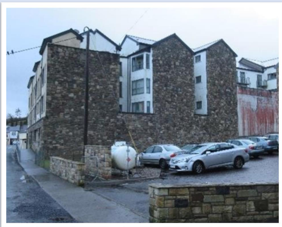
Fig. 52 Apartments & parking lot, Quay Road, Newport, 2018
