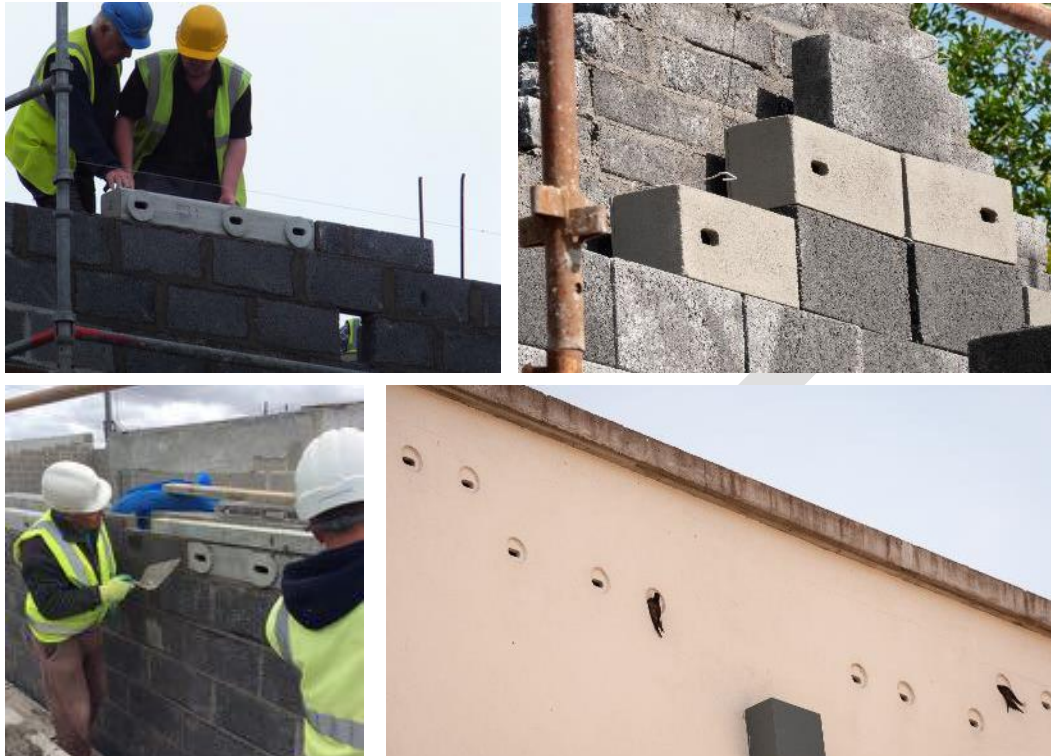
Plate 62: Swift nesting boxes can be easily incorporated into concrete block walls of buildings (images courtesy of Swift Conservation Ireland)
