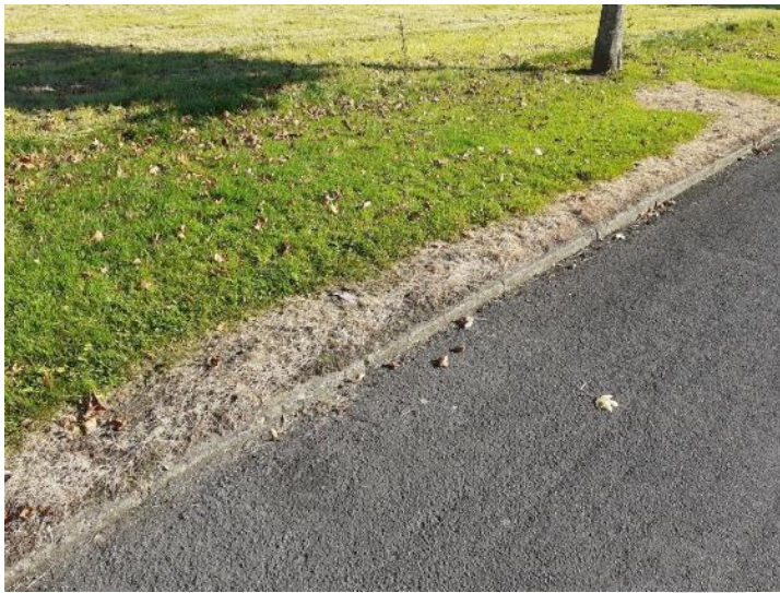
Plate 43: Here, weedkiller has been used unnecessarily along the edge of the road
