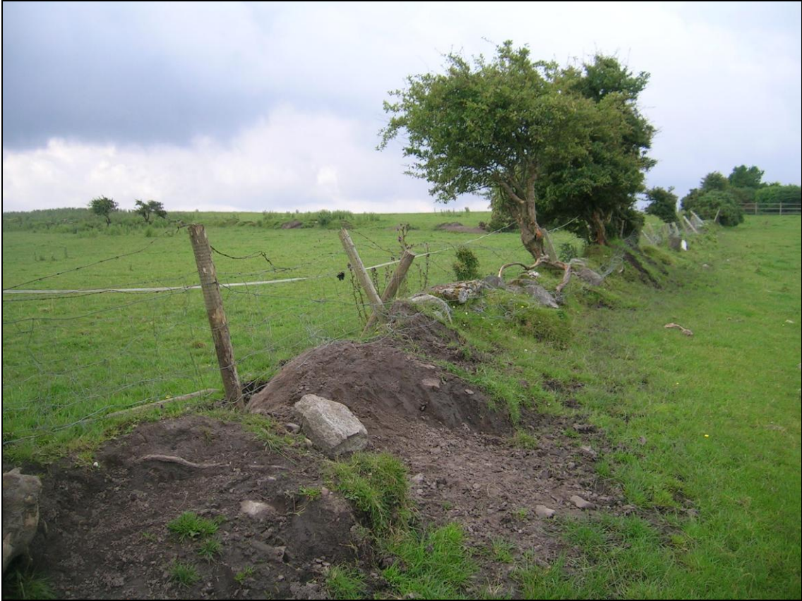
Severe degradation to Crossmolina (MO17) hedge bank
